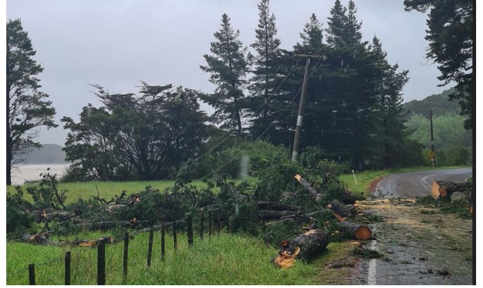
Photograph 4: Line damage in Tiniroto caused by trees outside the fall zone in November 2022
