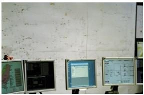
The SCADA system is used for real-time monitoring and control of the network. Frequency Voltage Current and temperature information is obtained from remote sites, and stored at 30 minute intervals. This information is used to report load trends for planning and alert operations staff of abnormal conditions.
