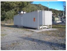
ENL purchased 6  $\times$  1.25MVA Diesel Generators in 2002 that supply at 11kV and include TOU metering. The units are capable of being relocated as required.
