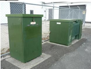
The distribution switchgear associated with the underground distribution network substations is predominantly ABB SD series Oil filled switchgear or ABB Safeplus SF6 gas filled switchgear. Switchgear installations are pad mounted and either located adjacent to or a short distance away from the substation installations.
